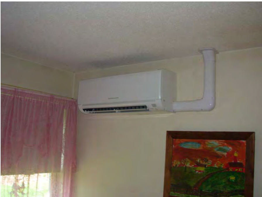
15. Unit heat pump HVAC system wall pack, typical Broder Place • Capital Needs Assessment • © On-Site Insight
