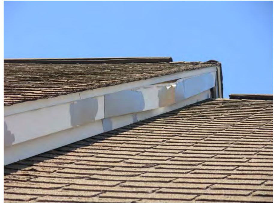
6. Spot trim element damage
