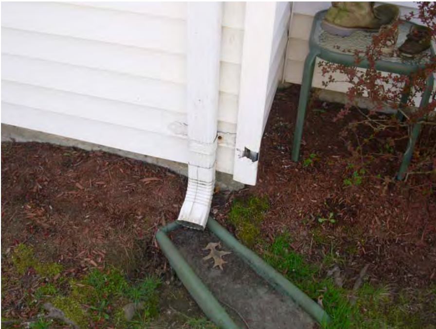
7. Spot vinyl siding damage, mostly at grade level
