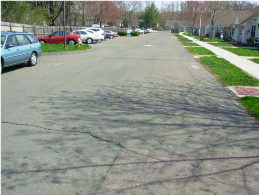
1. Sporadic cracking at parking, note newer walks
