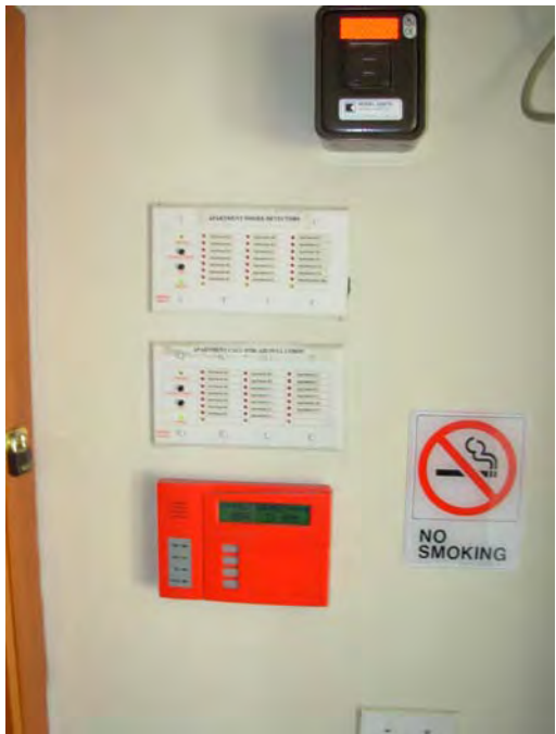
9. Fire detection - monitoring system panels
