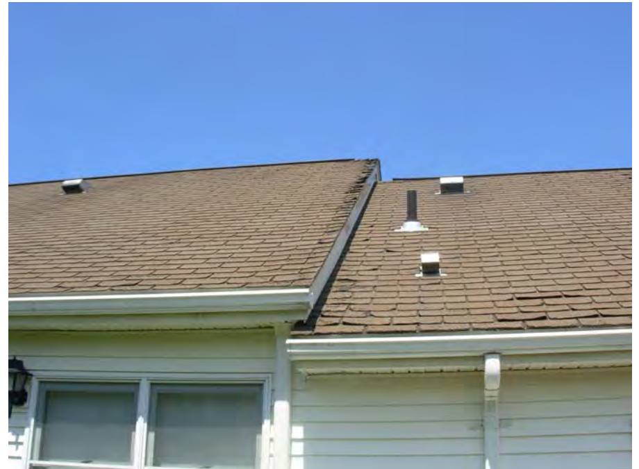
8. Lifting and curling of roofing shingles
