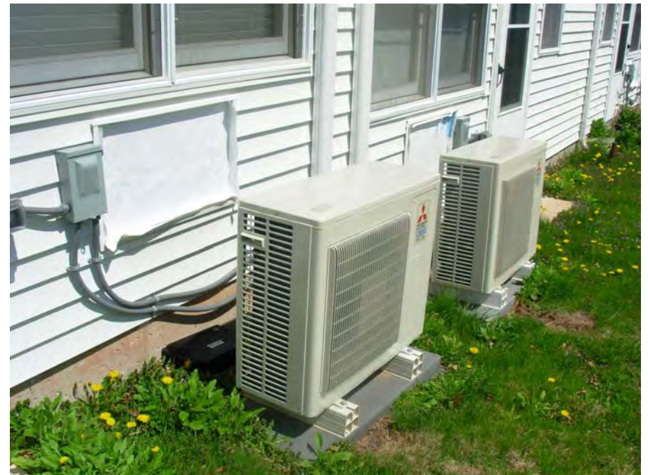
16. Heat pump HVAC system condenser units, typical
